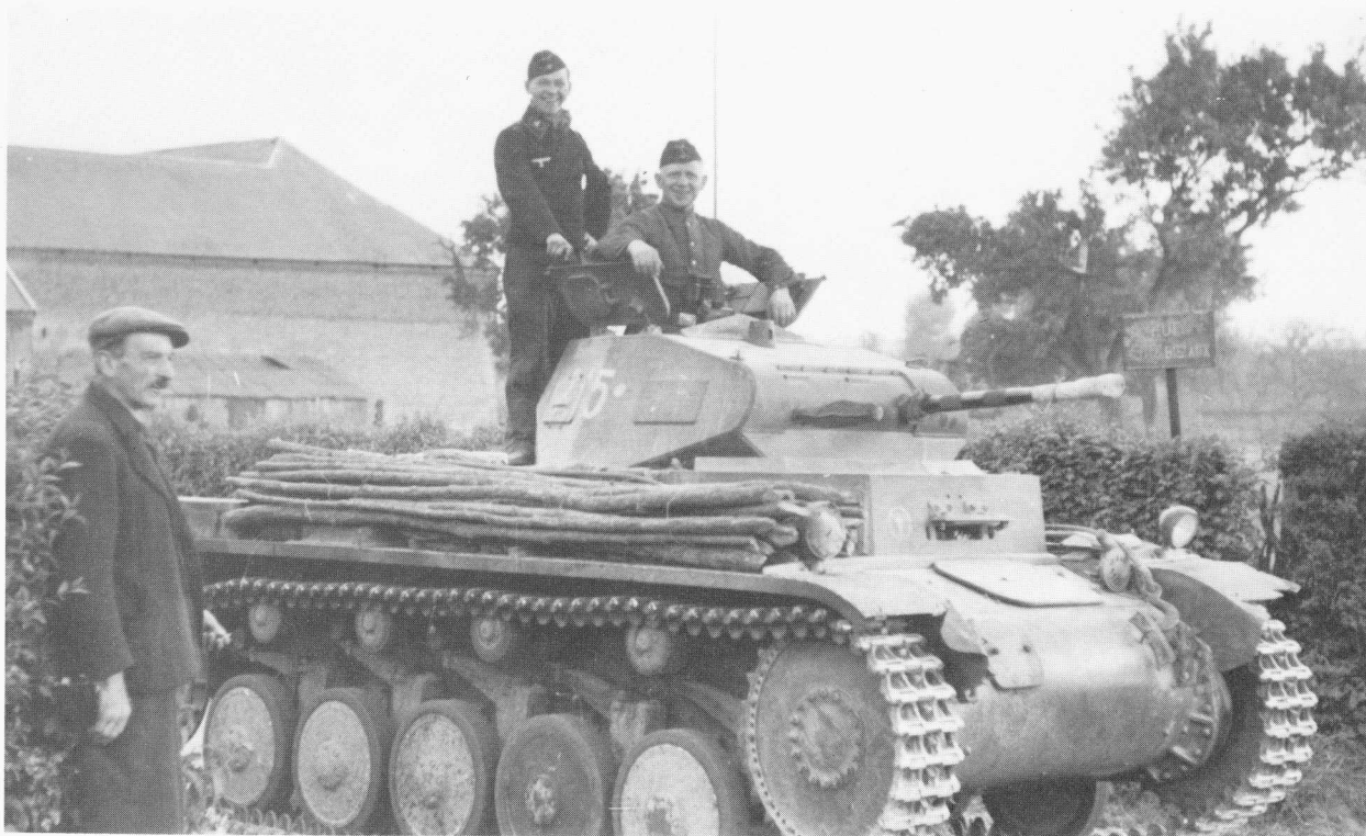
PzKpfw II Ausf. B of Pz-Regt. 36, 4. Pz-Div. in France, 1940. The Ausf. C was the last model to be produced with the original thinly-armoured, rounded bow. Experience in Poland showed it to be vulnerable even to anti-tank rifle fire, and eventually many of the early models were retrospectively fitted with a squared-off appliqué armour kit similar in appearance to the later variants. (US Nat. Archives)
