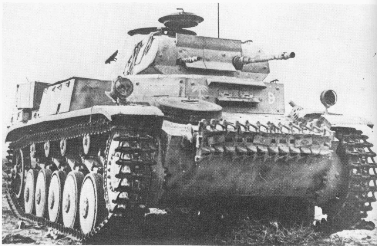
Fully up-armoured Ausf. A, B or C photographed in North Africa, with insignia of the Deutsches Afrika Korps and 21. Pz-Div. clearly visible. Note large bolt-heads, confirming the application of extra plate to the hull and turret front; the reinforced mantlet with 'splash' plates; and the angular bow. (RAC Tank Museum)
